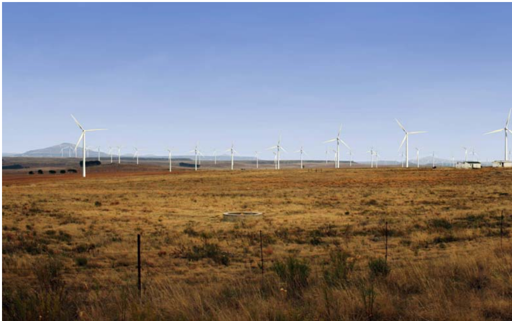
Figure 9.8: View west from R397 as it runs through the proposed facility, approximately 10km north-west of Sterkstroom. This view is indicative of what will be seen from the access gate of the farm Uitkyk.
